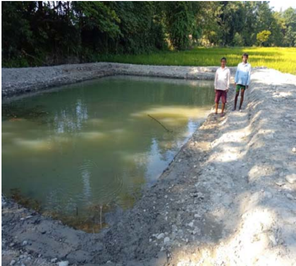
Farm Pond by MGNREGS (12.2M x 18.3M x 2.75M)
