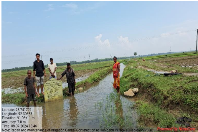
Canal construction through MGNREGA
